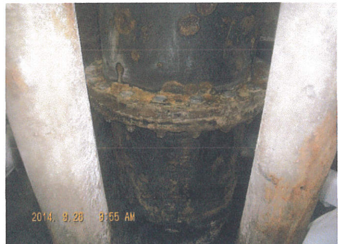
④ Next to the upper part of the pipe, carry out descaling at the lower part.
