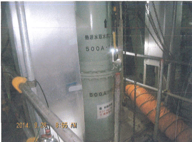
①check the repair site.
