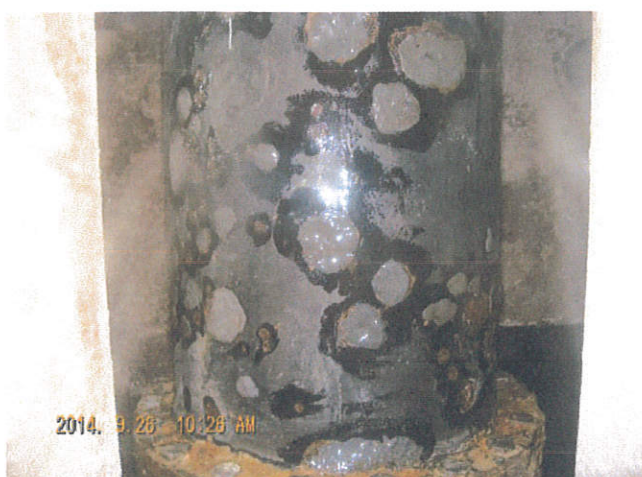
⑤First, fill the Magicawrap-Steel over the uneven part
